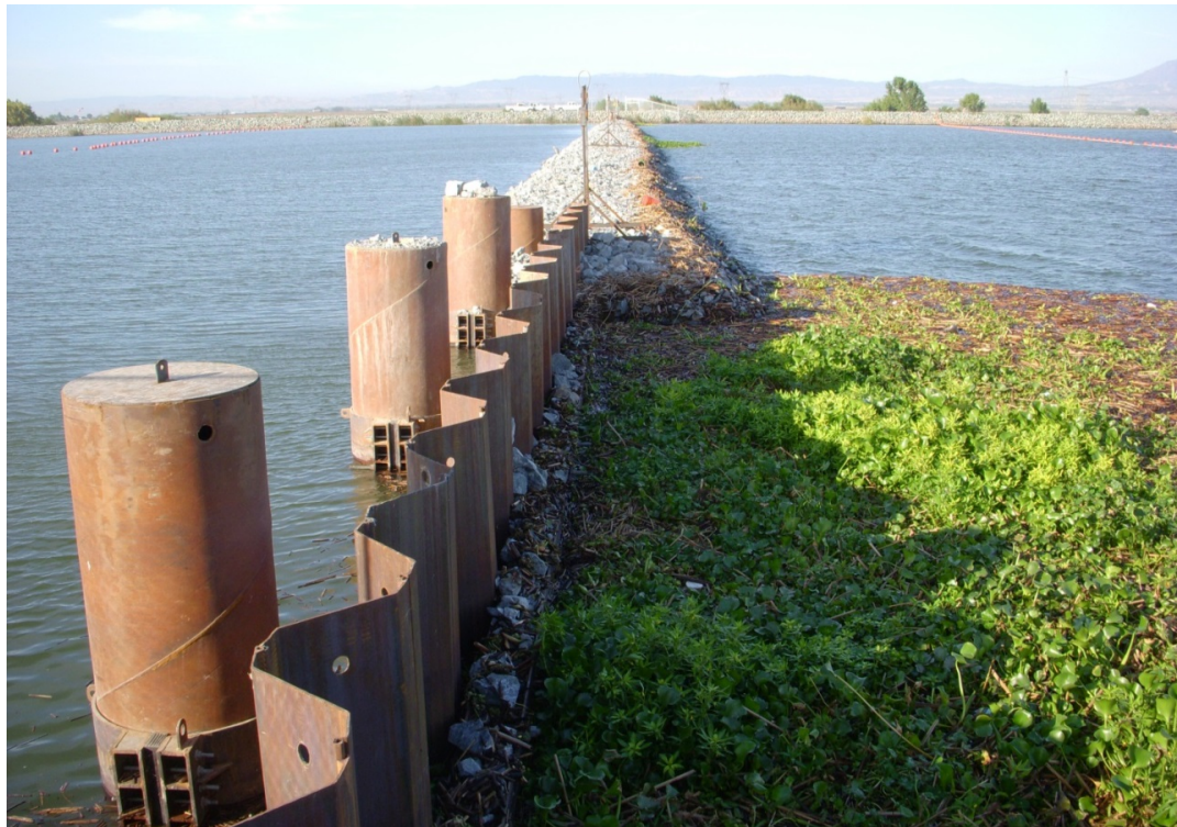
Photo 2: Completed barrier, looking south from Bradford Island to Jersey Island (June 17, 2015).
